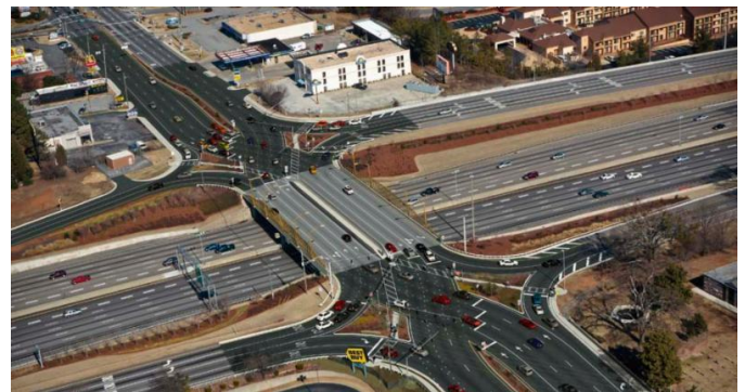
I-85 and Pleasant Hill Road Diverging Diamond Interchange
