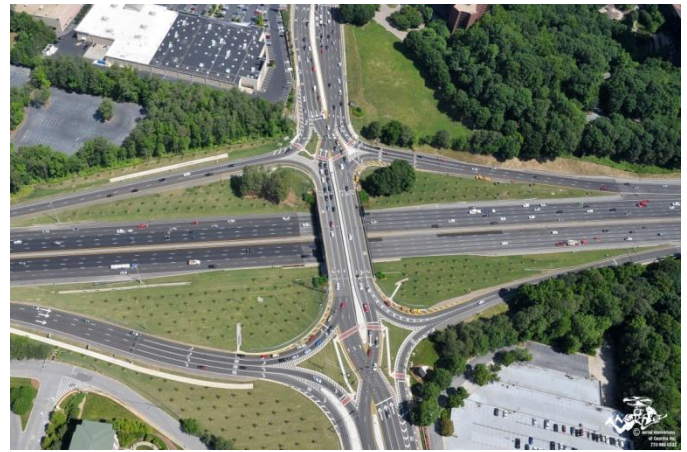
I-285 and Ashford Dunwoody Road Diverging Diamond Interchange
