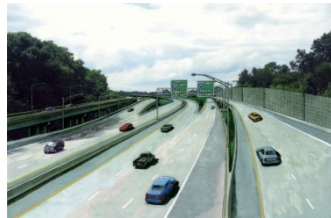
I-16 Westbound with extended noise barrier
